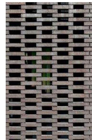
5 Perforated Brick Detail
